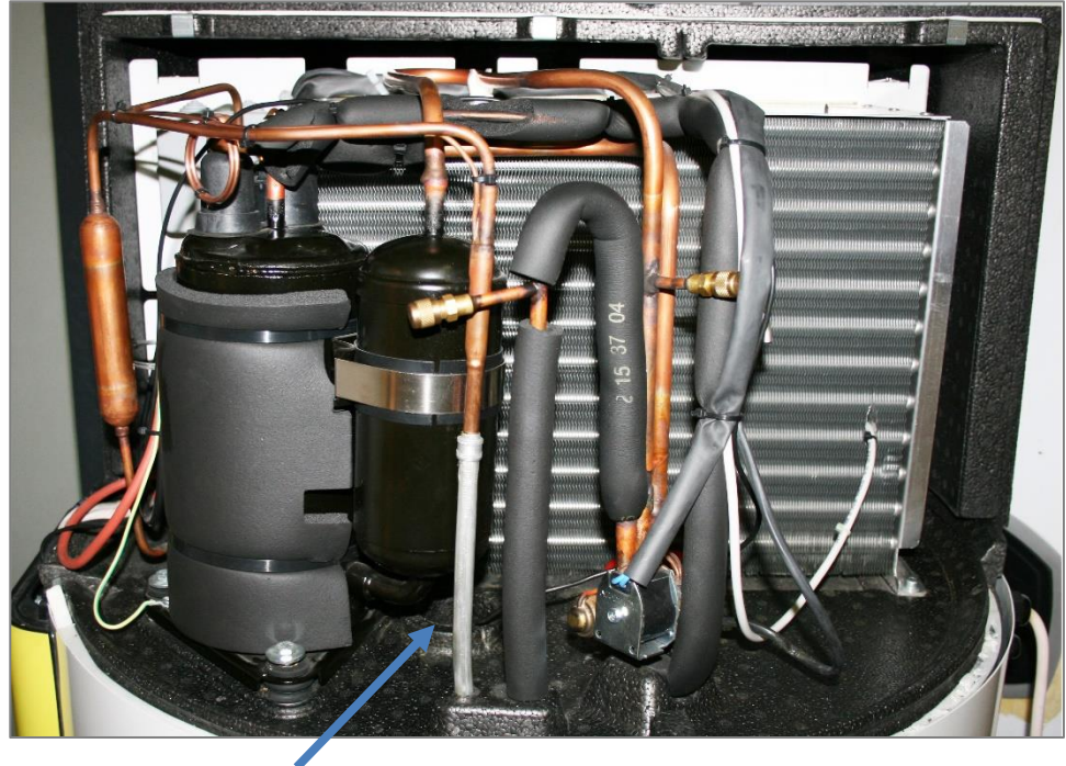
Figure 18: Position magnesium stick (see arrow)
